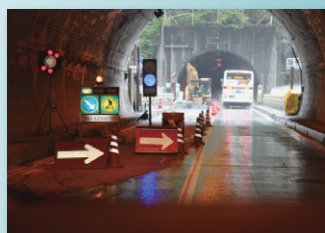
Service and utility tunnels, construction sites
